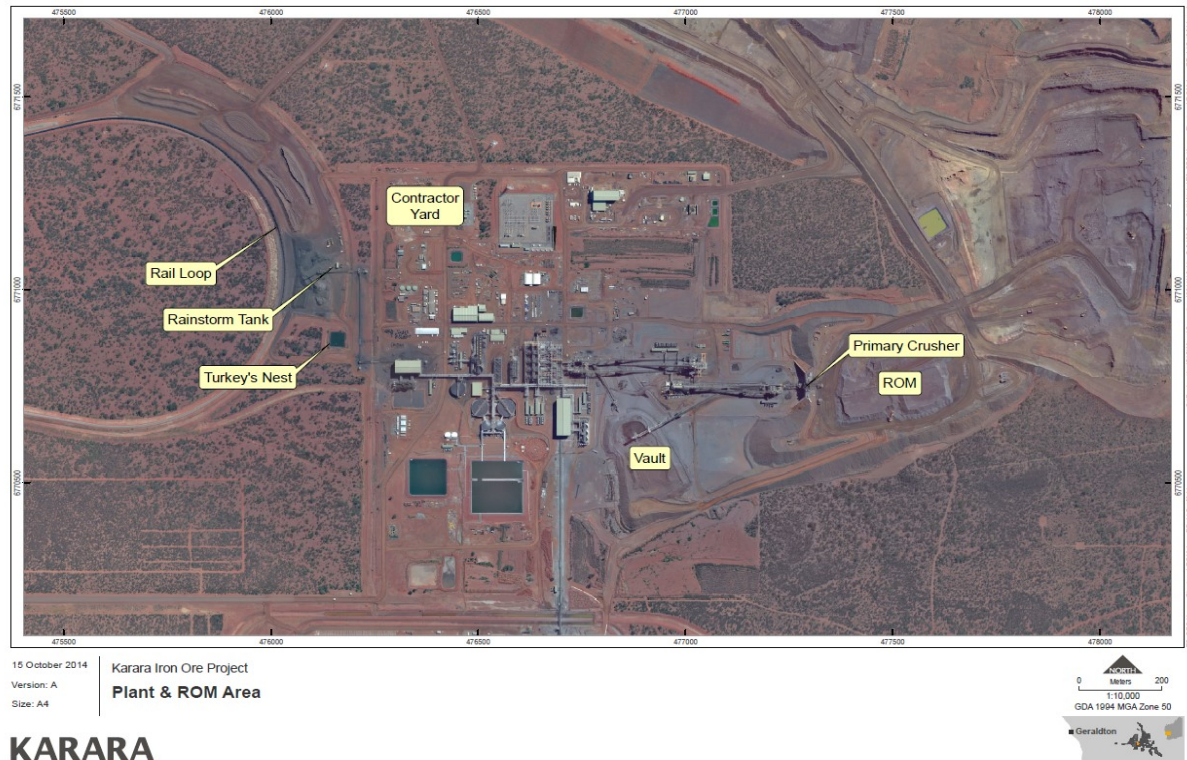
Figure A: Karara Mining Limited Plant, ROM and Rail Train Loadout Overview.
