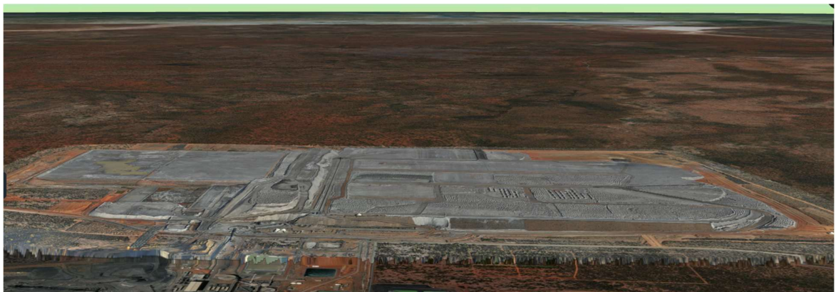
Figure 7: TSF Looking SOUTH
