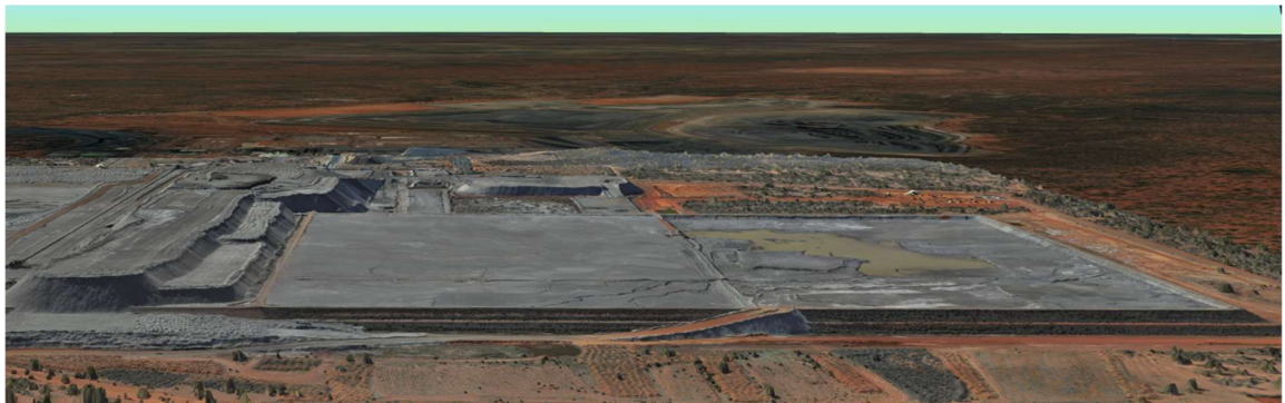
Figure 6: TSF Looking NORTH
