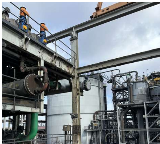
Figure 42: Installed DN600 Valve
