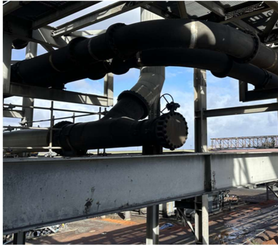
Figure 43: Installed DN600 valve
